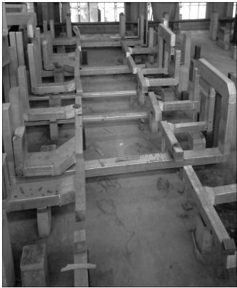
图 8 静流式电解槽母线现场施工图 Fig.8 Construction site of stationary stream pattern pot
