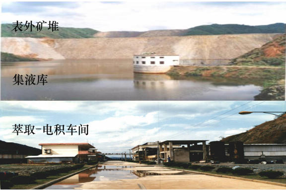
图 15 江西德兴铜矿微生物冶金工业应用 Fig. 15 Application of biohydrometallurgy in Dexing copper mine, Jiangxi province
